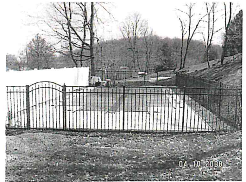
Figure 4. Inground swimming pool completely enclosed by fencing.
